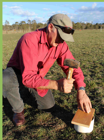
3- Hammer in the PVC tube using a block. Make sure it is level and firmly in the ground.
